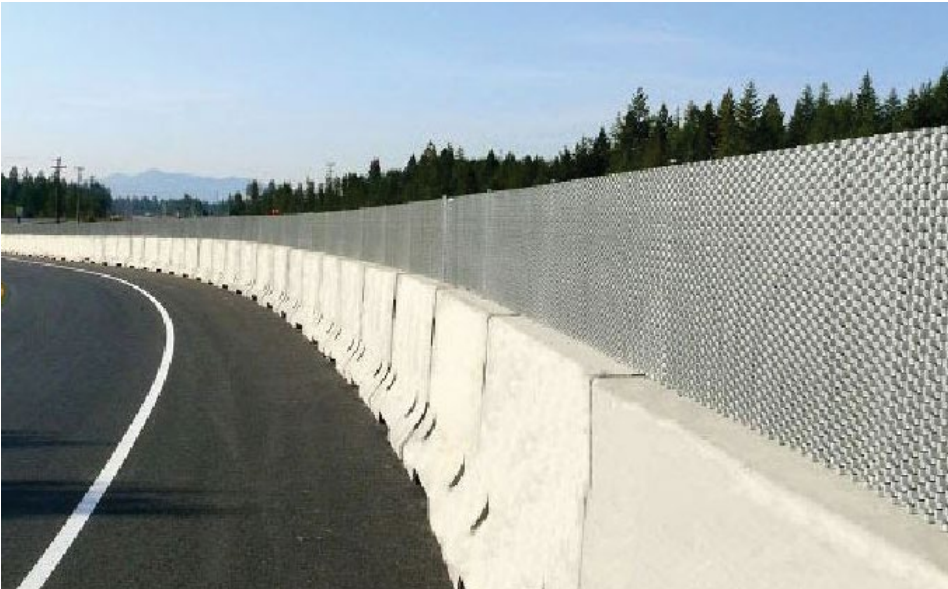
Figure 93: Example image of Retaining Wall with Anti-glare Screen on top
