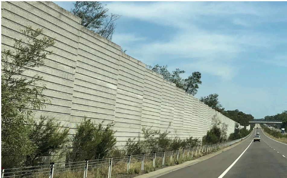
Figure 84: Typical noise wall arrangement from Hunter Expressway to be considered for Noise Wall Type 3
